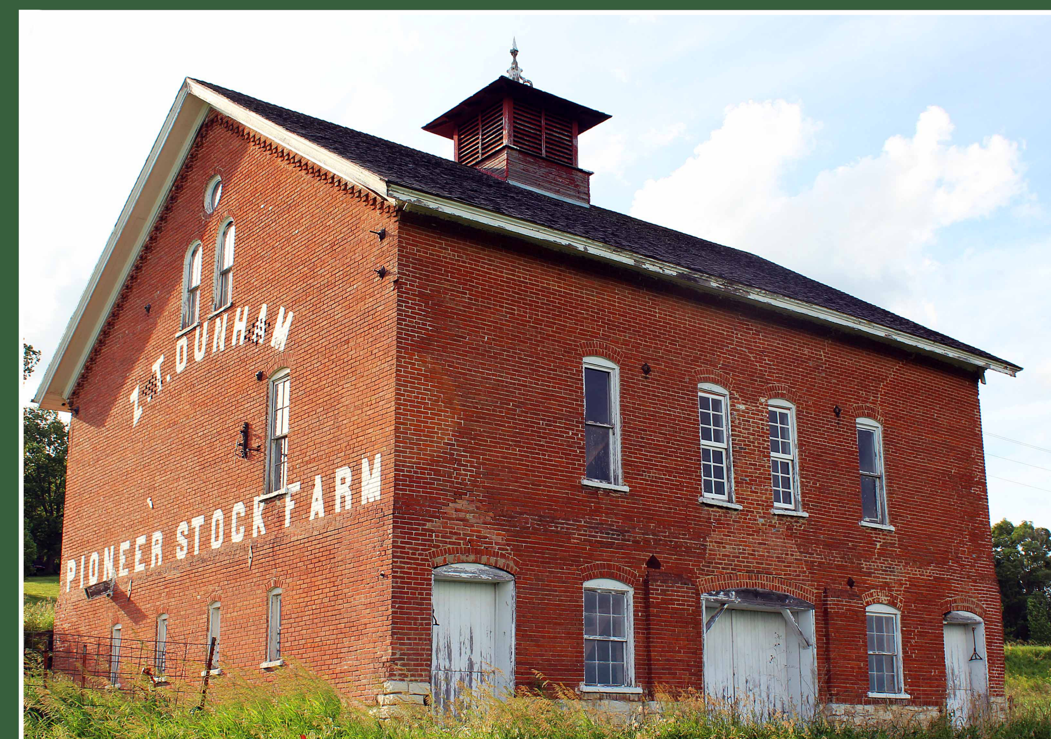
In 1981, Virginia Dunham initiated the procedure to get the barn on the National Register of Historic Places.
